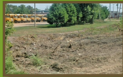
Clean-out at Rosa Fort High School has helped prevent flooding at the school.
